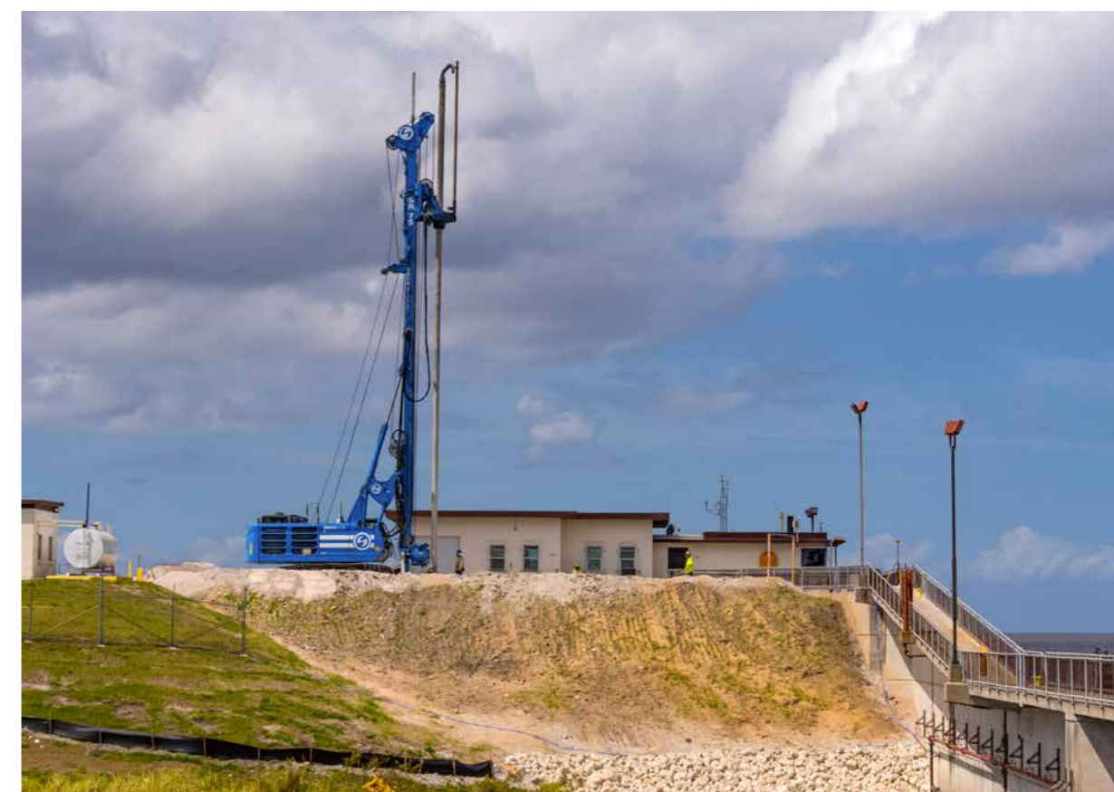
Rehabilitation of Herbert Hoover Dike, Florida, USA
