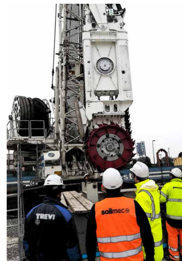
TTMJ: Test field, Cesena, Italy
