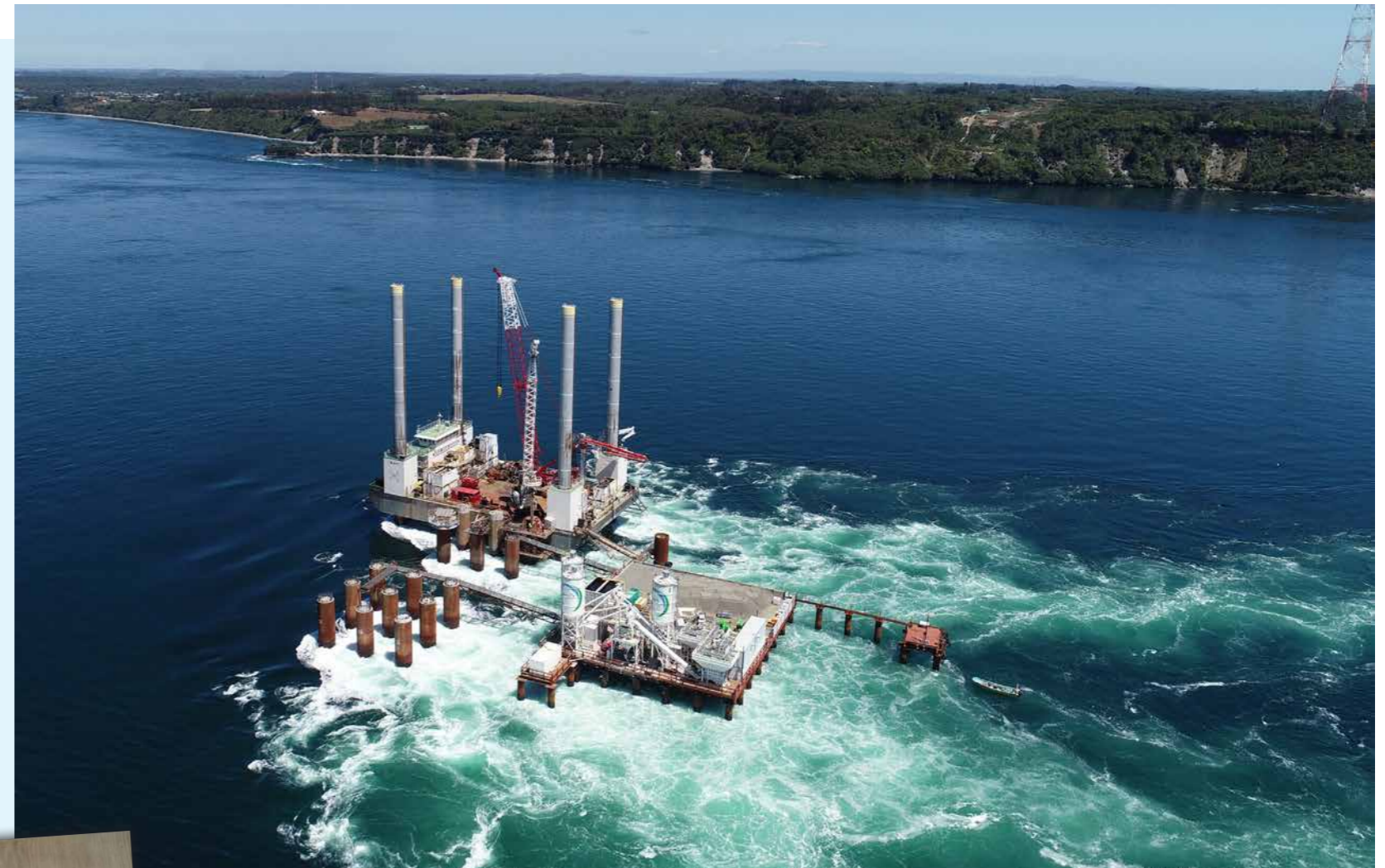
Chacao Bridge, foundation works for pylon number 1_Chile
