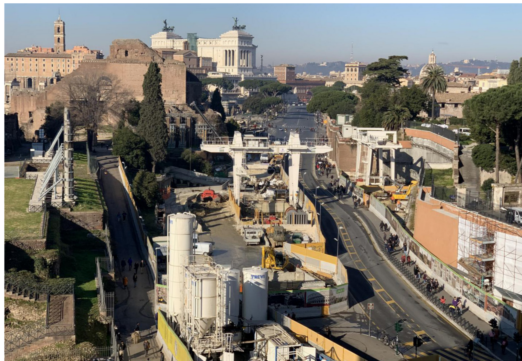
New line "Metro C", station of "Fori Imperiali", Rome, Italy
