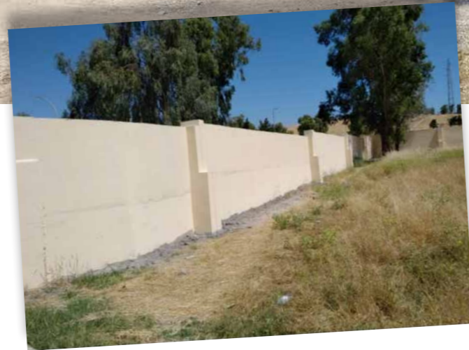
New surrounding wall of the high school for girls in the village of Mosul.
